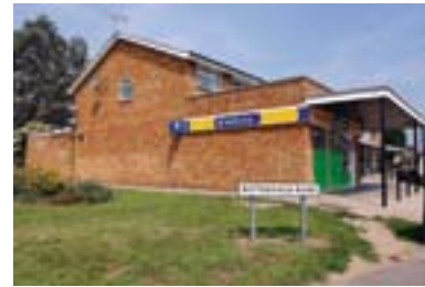
The dead wall at the end of the parade of shops could be improved by landscaping the small green, including planting several native trees.
