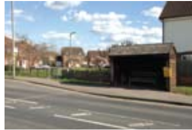
Bus passenger shelter in Main Road.
