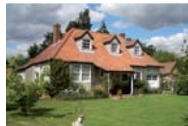
An example of dormer windows.
