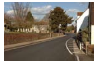
The low brick walling alongside the church.
