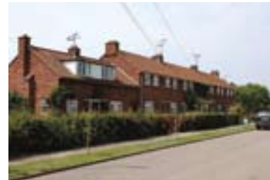
Terraced council built housing in The Chase.
