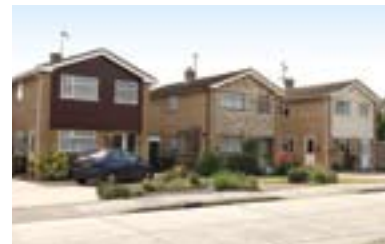
Link-detached houses in Juniper Road.
