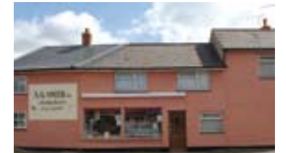
The Village Butchers blends well with the surrounding houses.
