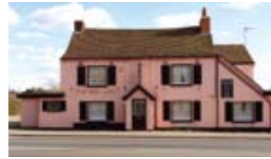
The Red Lion — Currently being redeveloped as a pub, hotel and restaurant.
