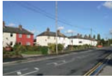
Oak Cottages along Main Road.
